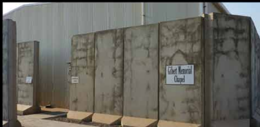
>> McCormick’s unit attends Mass at a chapel surrounded by concrete blast barriers called T-Walls, which help to protect occupants from incoming mortars.
